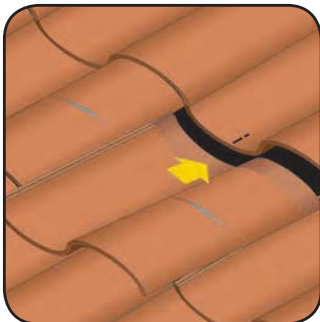
Step 9: Replace the tile by lining up the snap lines and mark the drill location accordingly.
